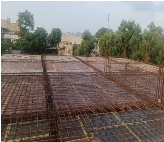
Steel mesh laid for the RCC roof slab, August 2025
