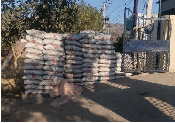
Materials procured directly by BSS for quality control
