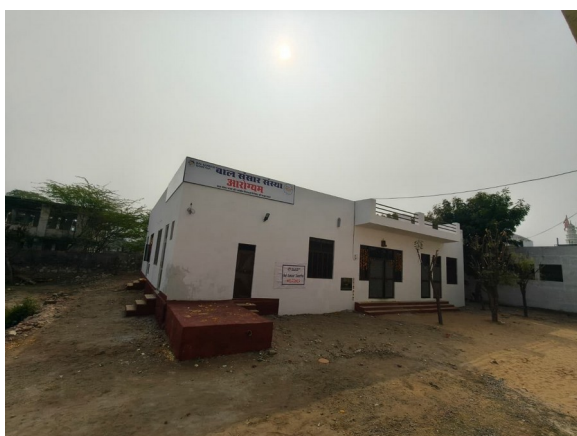
The completed Aarogyam Kendra, Hathikhhera campus
