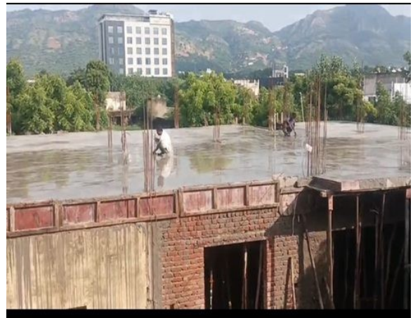
RCC slab cast and cured, September 2025
