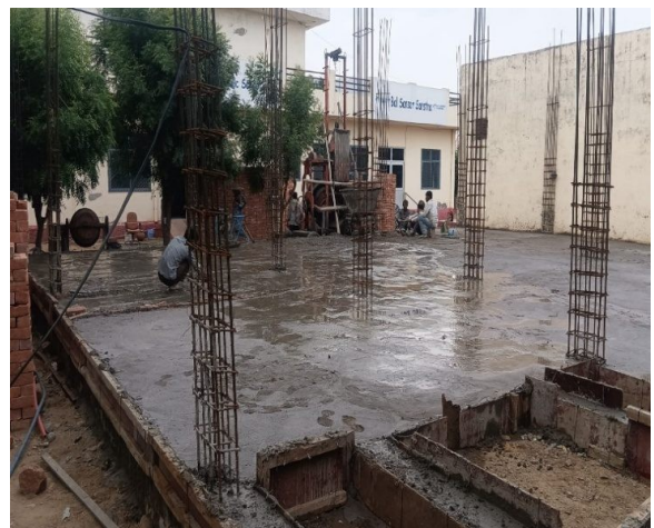
DPC / plinth level reached, May 2025
