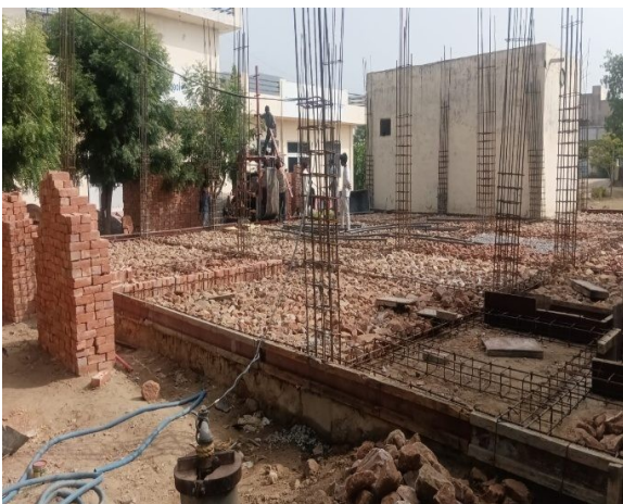
Footing and column work, April-May 2025
