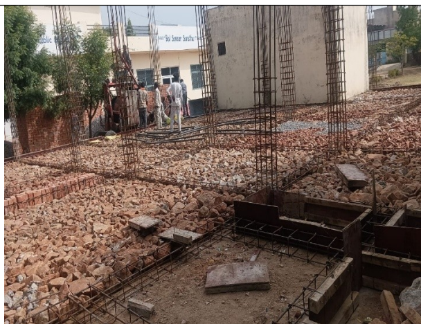
Plinth beam and column work in progress, April 2025
