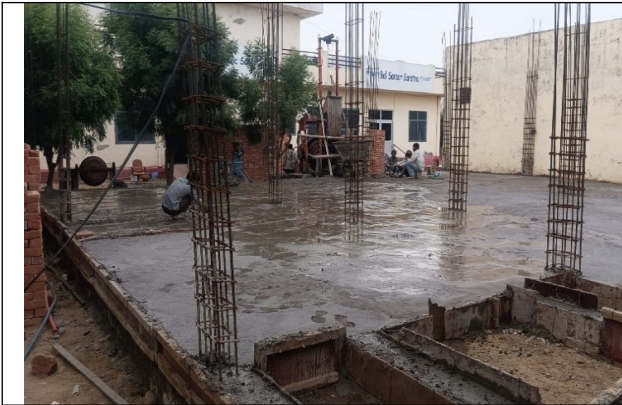
Ground floor RCC slab casting in progress, May 2025
