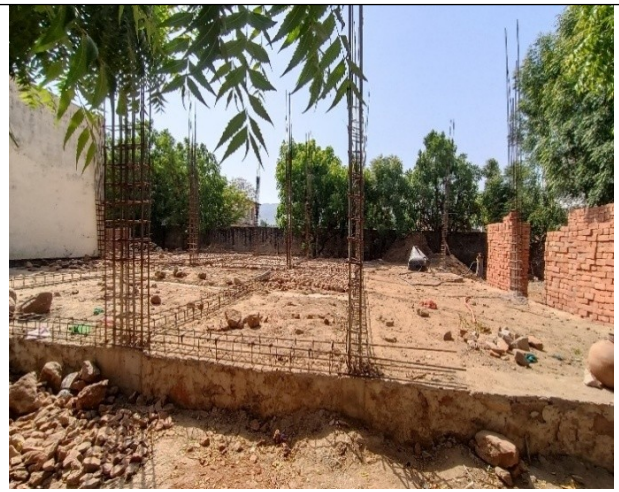
Column framework at early stage, March-April 2025
