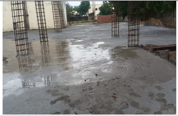
Cured slab with columns, May 2025
