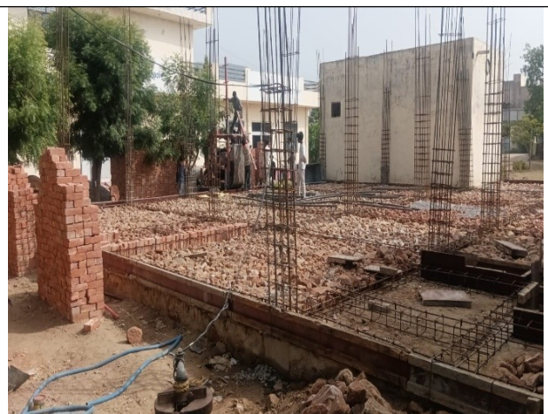
Column and brickwork rising, April 2025
