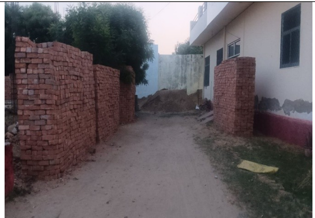
Boundary wall construction progress
